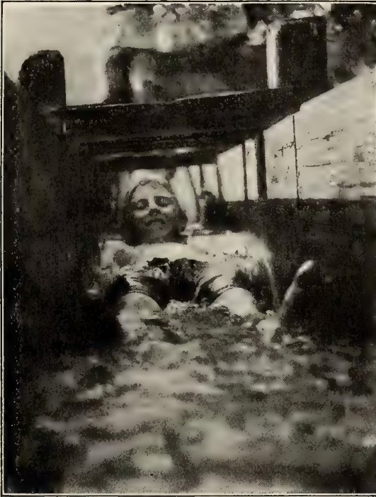
"CHUTING" A BOX-FLUME, FEET FOREMOST. (SEE NEXT PAGE.)
